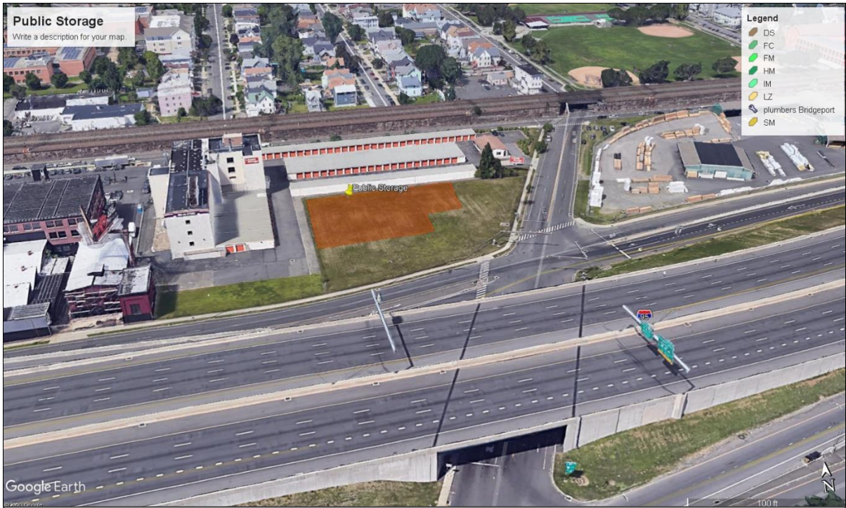
Figure 1: Google Earth Bird's Eye View
