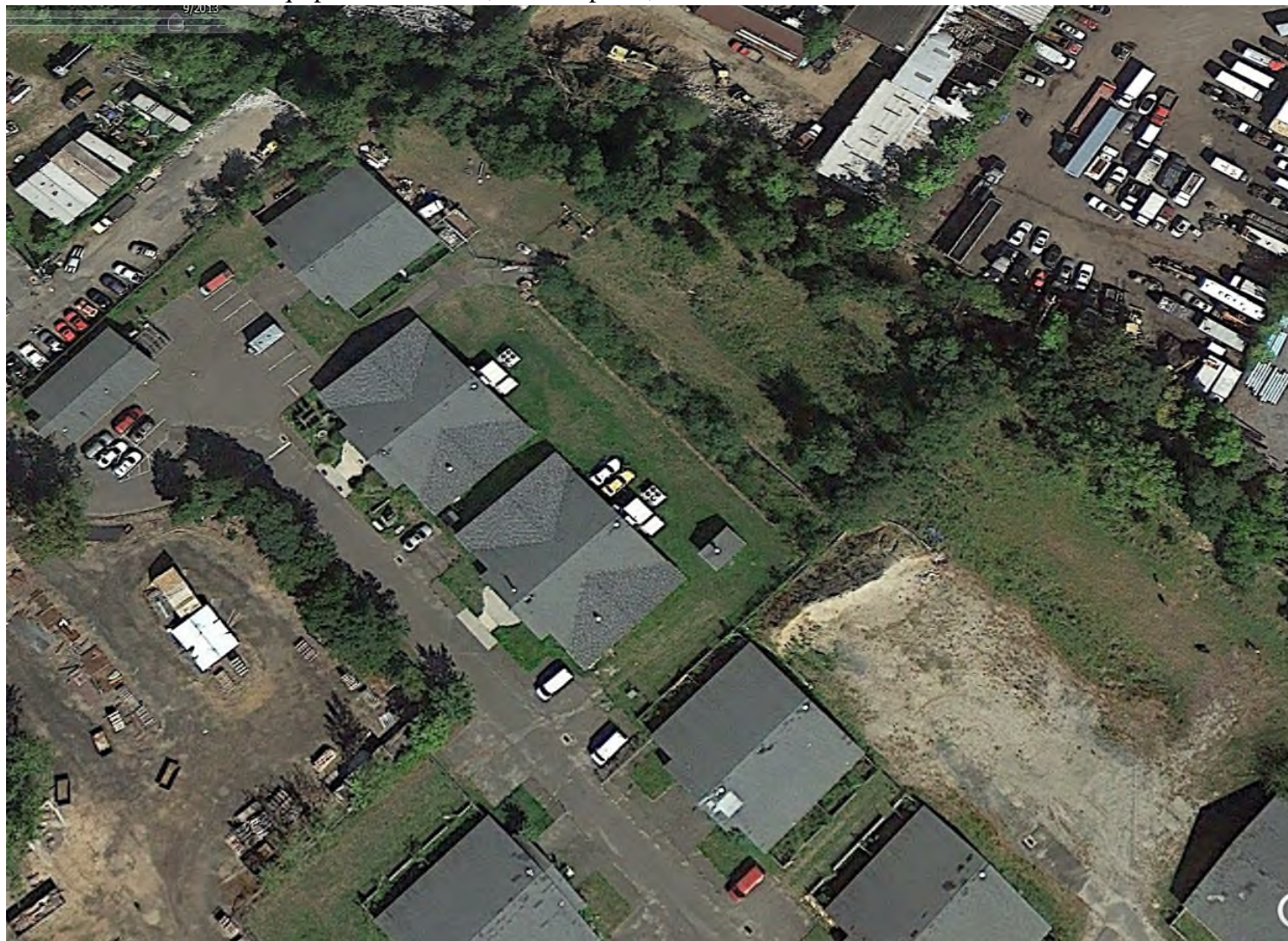
YR 2013-Construction equipment removed, trees in place, mound of dirt remains.
