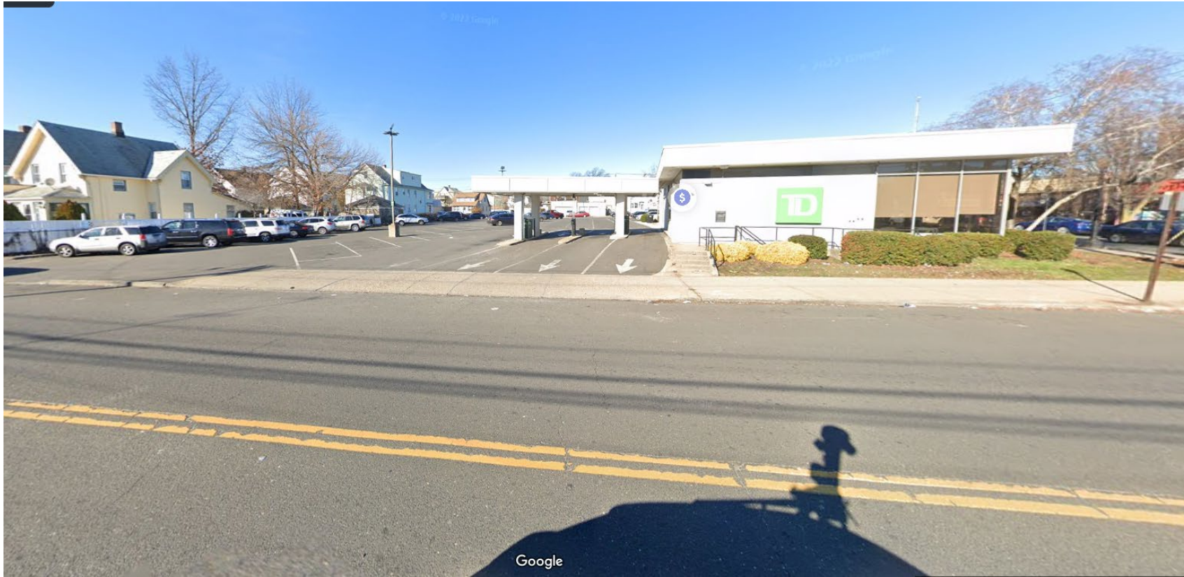
The Property from Capitol Avenue
